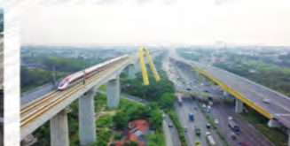
JAKARTA-CIKAMPEK ELEVATED TOLL
